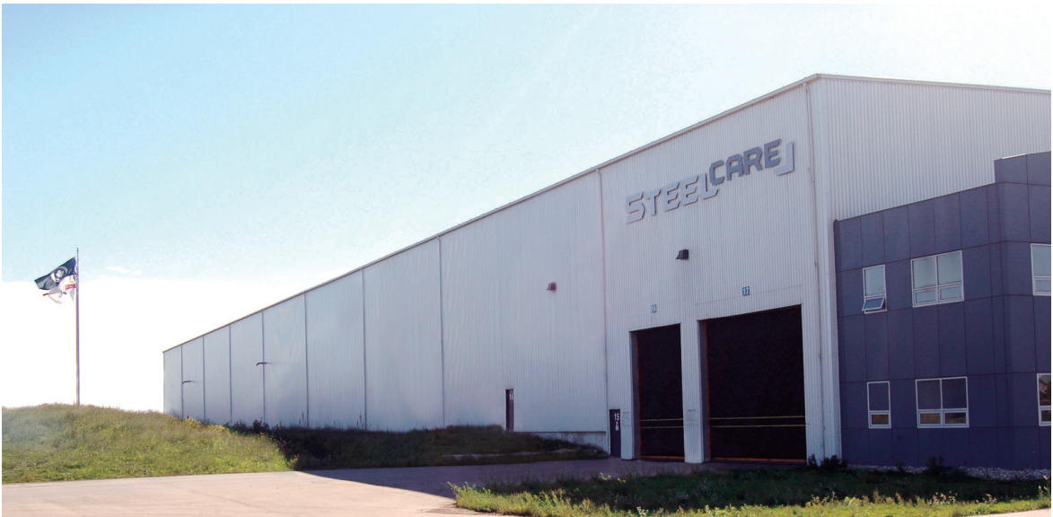
Figure 4-3. Exterior view of Steelcare, Inc.
